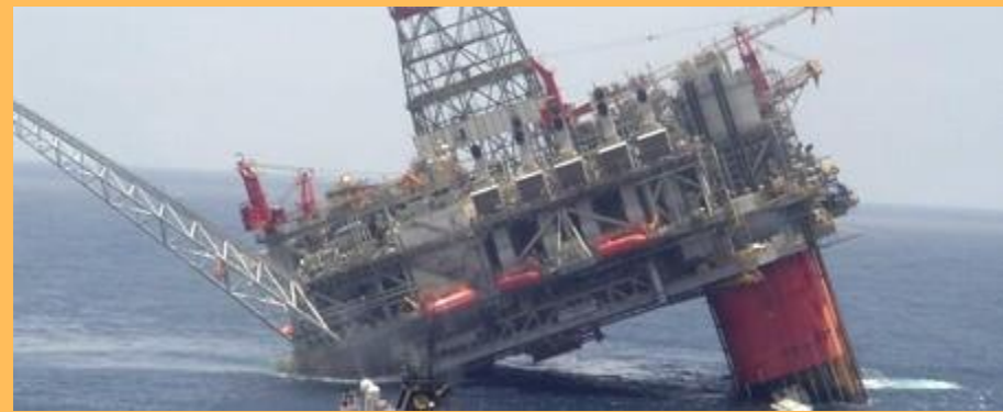
Thunder Horse platform after Hurricanes Katrina and Rita. It was just brought back online this year. Photo from MMS.
